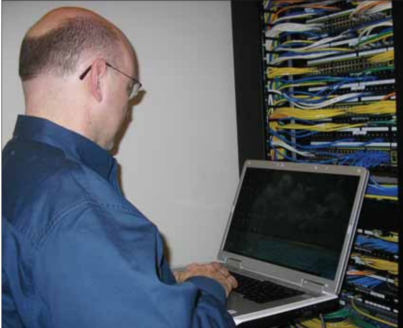
Greg Coon, service manager with ProTech Security of North Canton, Ohio, programs a fully IP-based security system that includes an S2 NetBox access control device using an ordinary LAN connection at Jackson High School.
